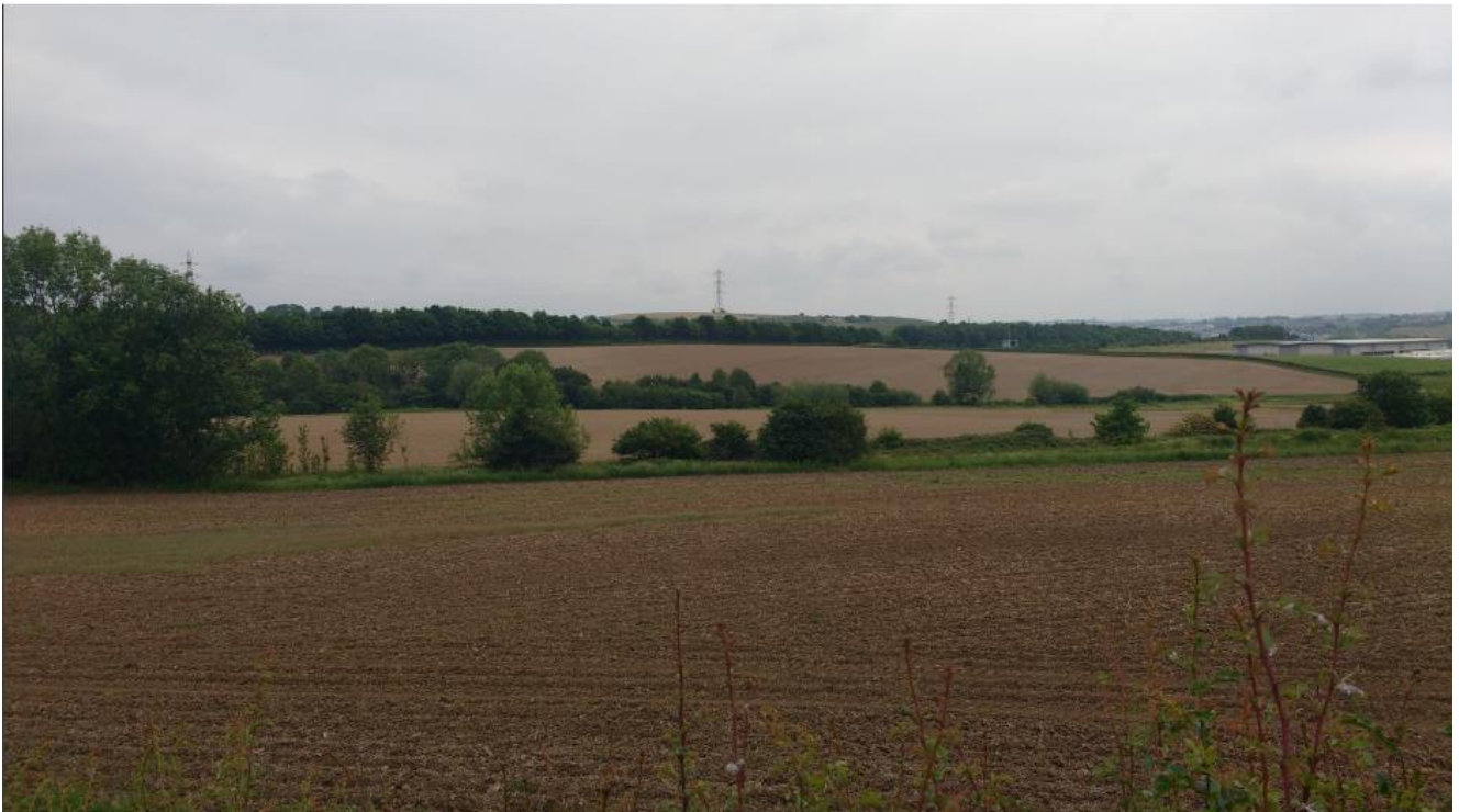
From the northern point of the site looking south across the Oxcroft Branch Line (foreground), then Hawk Brook river corridor valley, then site of Building A site raised above the level of the 'Gist' building (far right), then tree line to the M1 as horizon.
